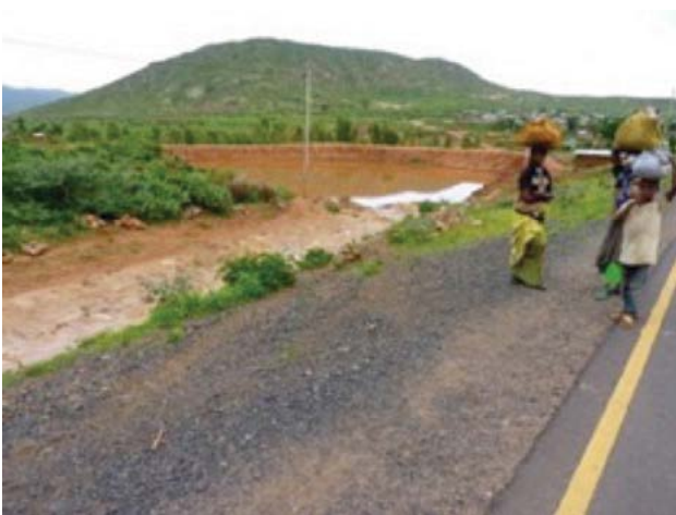
Figure 14: A pond collecting drainage water from a road drains (Source: Francesco Sambalino).
